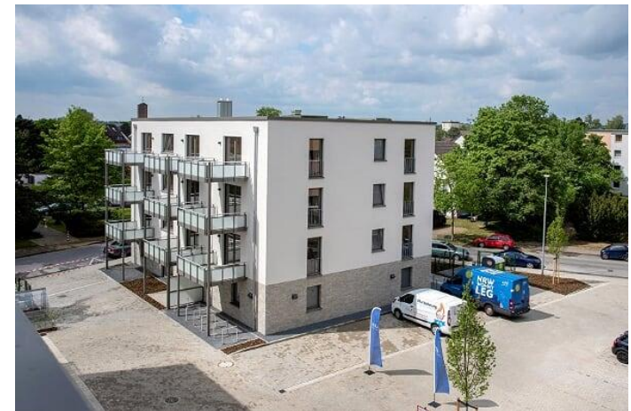
New construction in Hilden
