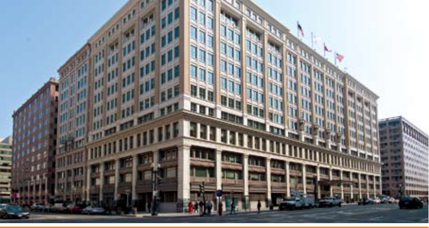
HOMER BUILDING, WASHINGTON DC, US
